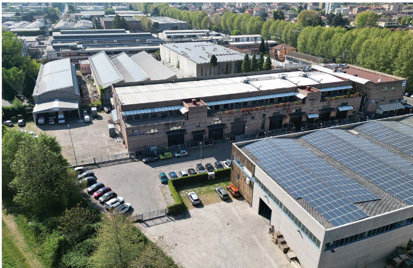
Brizio Basi plant 1 and plant 2 with energy autonomy
